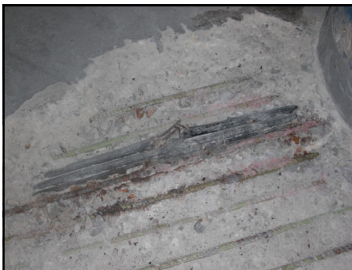
Exposed broken post-tension cable located at concrete de-lamination.
