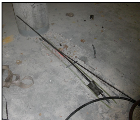
Repair of post-tensioned cable.
