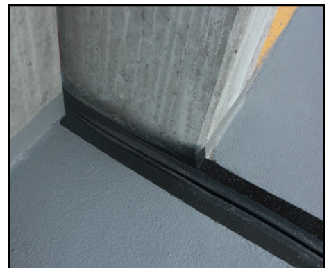
Detail of newly installed expansion joint.
