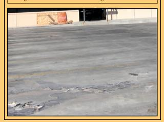
2.) Moisture gets in to cracks and starts breaking down the concrete, causing rusting on reinforcing steel, post tension cables and jeopardizes the structural integrity.
