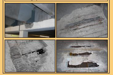
3.) The correct recourse to mitigate this type of destruction is to mechanically remove the coating, remove spalled concrete, repair reinforcing steel and post tension cables, replace the concrete, route and caulk control joints, and properly re-install a waterproof membrane system.
